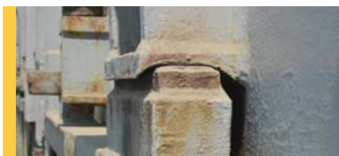
WORN OUT MATING SURFACE OF A BEARING PAD.
