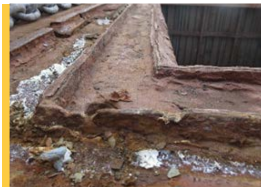
HEAVILY CORRODED AND DAMAGED COMPRESSION BAR.
