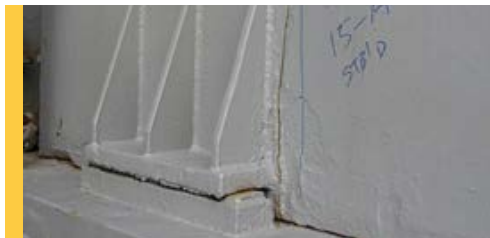
CRACKED PANEL SIDE PLATING AS A RESULT FROM WEAR ON BEARING PAD.
